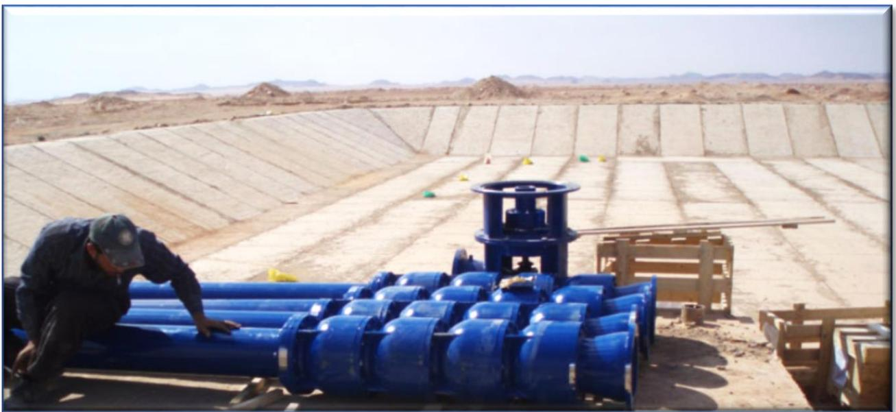
In the picture on the right is shown the hydraulic part of the 22" pump in the phase of installation into the well.
