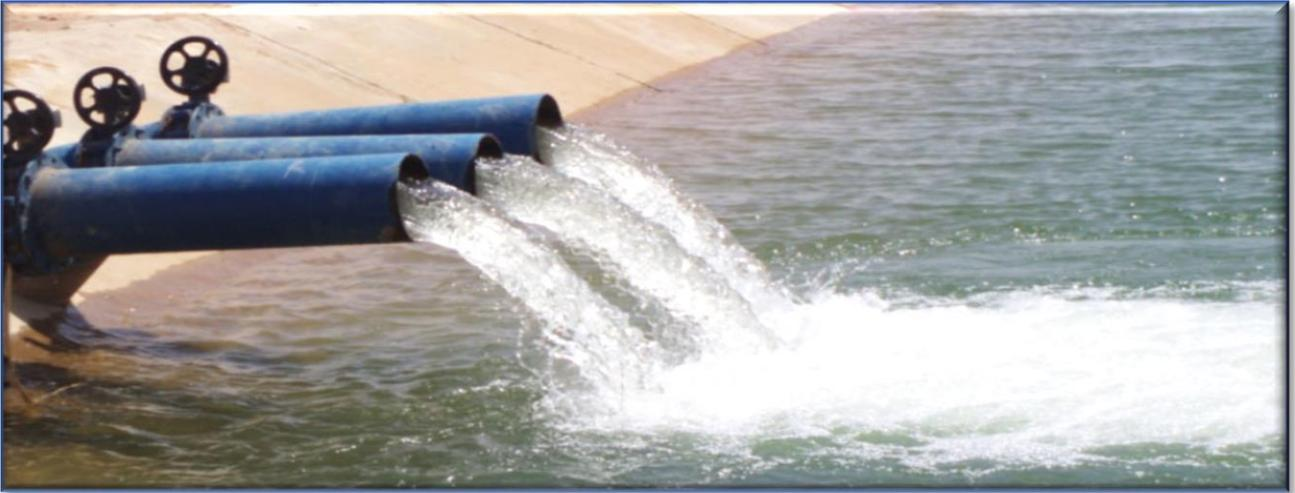
In that picture is shown the booting pumps, which suck the water from the basing to feed the pivot irrigation systems.
