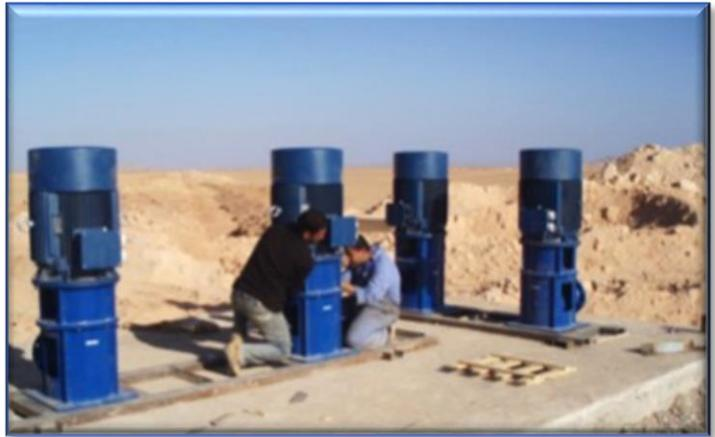
In the following picture is shown the preparation phase of the collection water basin which will be fed from the said 30 vertical turbine Marly pumps.
