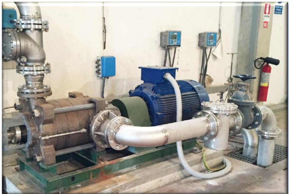
Below picture shown a Marly pumping station made of 3 End-Suction pumps model CAX150-400 with 75Kw motor and 2 multistage pumps model HPR 125/5 with 90Kw motors.
